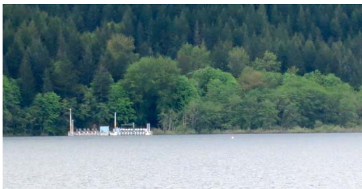
Figure 5. Anchored Floating Station
